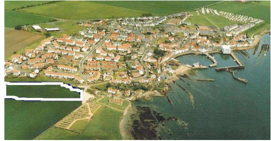
AN ARIEL VIEW OF ST.MONANS White line depicts boundary of proposed site
