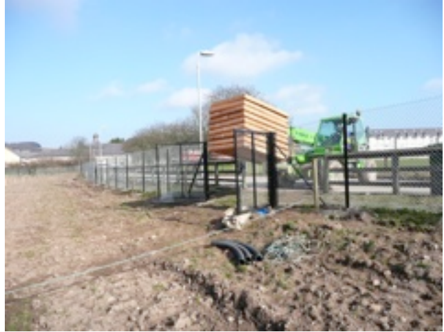
The fence, main gate and a shed delivery, March 2011
