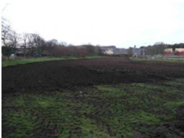
Breaking ground, February 2011
