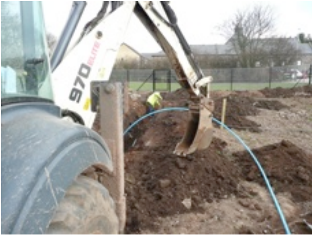
Installing a mains water supply, March 2011
