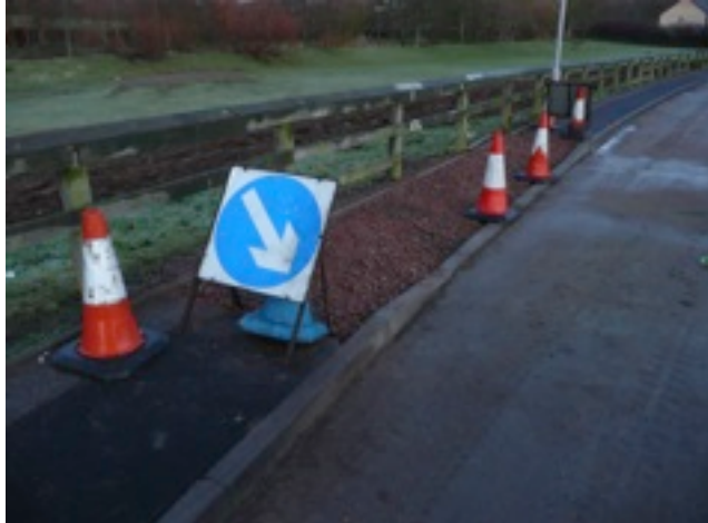
Dropping the kerb for the main gate, February 2011
