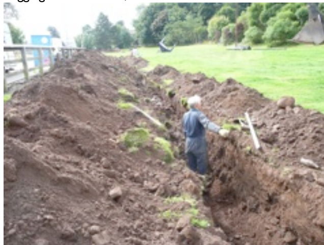
Digging the land drain, Autumn 2010
