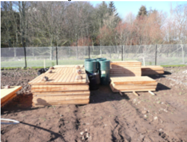
Sheds and rainwater goods, March 2011
