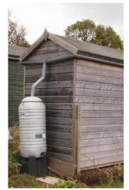
This proprietary water butt system connects to the gutters. Works on double pitch roofs, 200L butt shown. Bridgend Farm, Edinburgh
