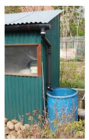
A DIY water butt collects the water from a plastic gutter. The single pitch of the hut minimises infrastructure. Mansewood, Glasgow
